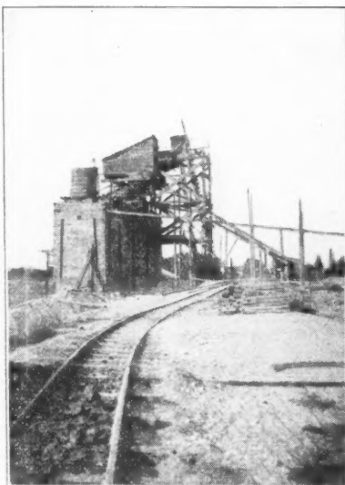
The Screening and Washing Plant.
